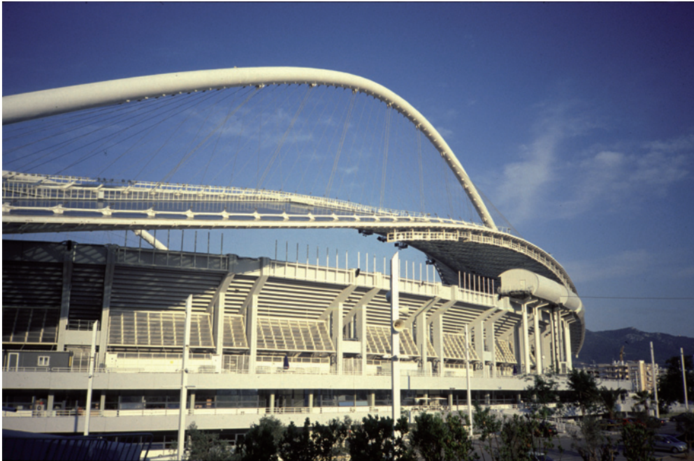
Figure 5.3 In the 2004 Olympic Stadium in Athens the structure is visually dominant. Architect: Santiago Calatrava.
