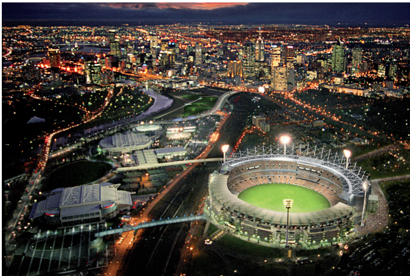
Photograph: HOK Sport Architecture
