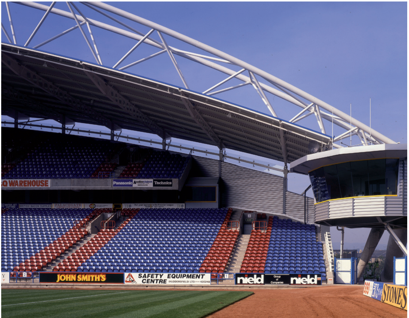
Figure 19.2 The control room at Galpham Stadium, in Huddersfield, is located to give a clear view over the playing field which cannot be obstructed by, for instance, spectators.
