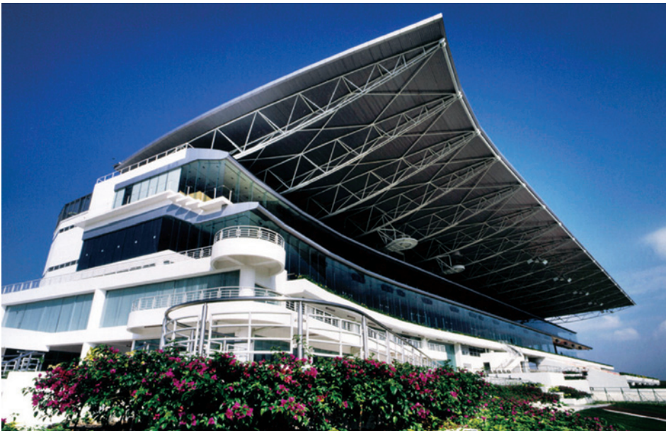
Figure 5.10 The cantilevered roof at Selangor Turf Club, Malaysia, is mainly designed for protection from the sun. Architects: T. R. Hamzah & Yeang Sdn. Bhd in association with HOK Sport Architects. Structural engineers: Tahir Wong.
