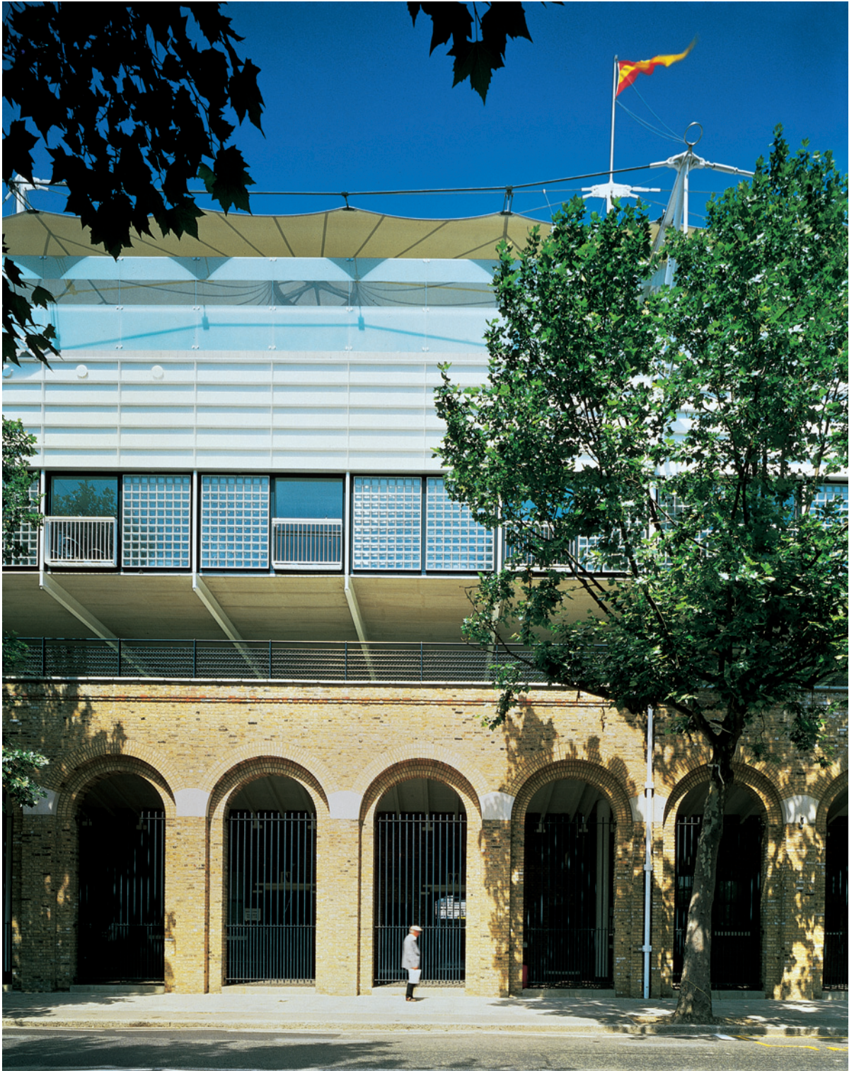
Figure 5.2 In urban contexts the most appropriate approach may be a dominant façade with the roof either hidden or subdued. The Mound Stand at Lord's Cricket Ground, London has a light roof floating above a dominant and well-composed façade. Architects: Michael Hopkins & Partners .
